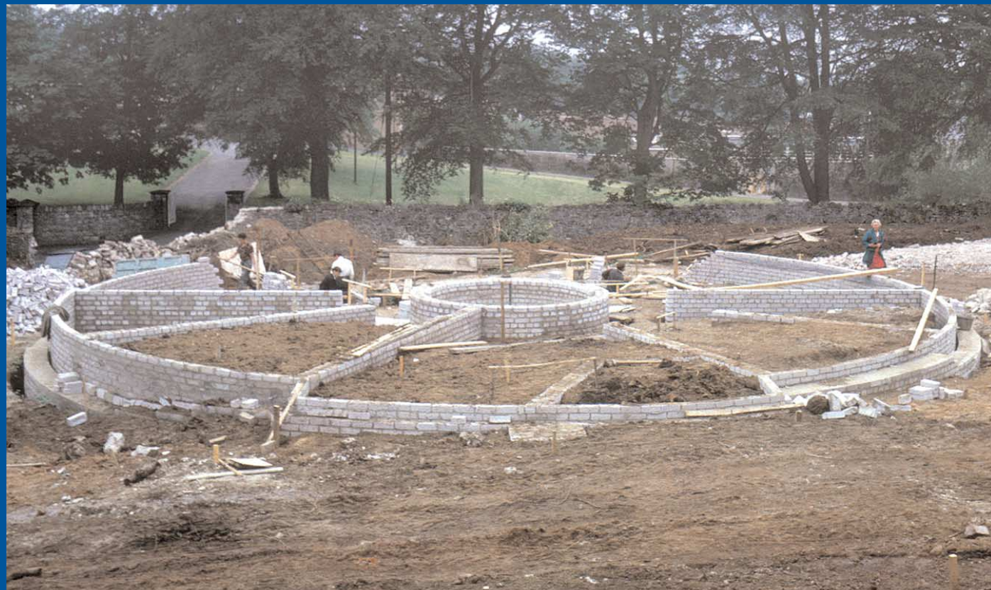
The foundations are laid: 1966
